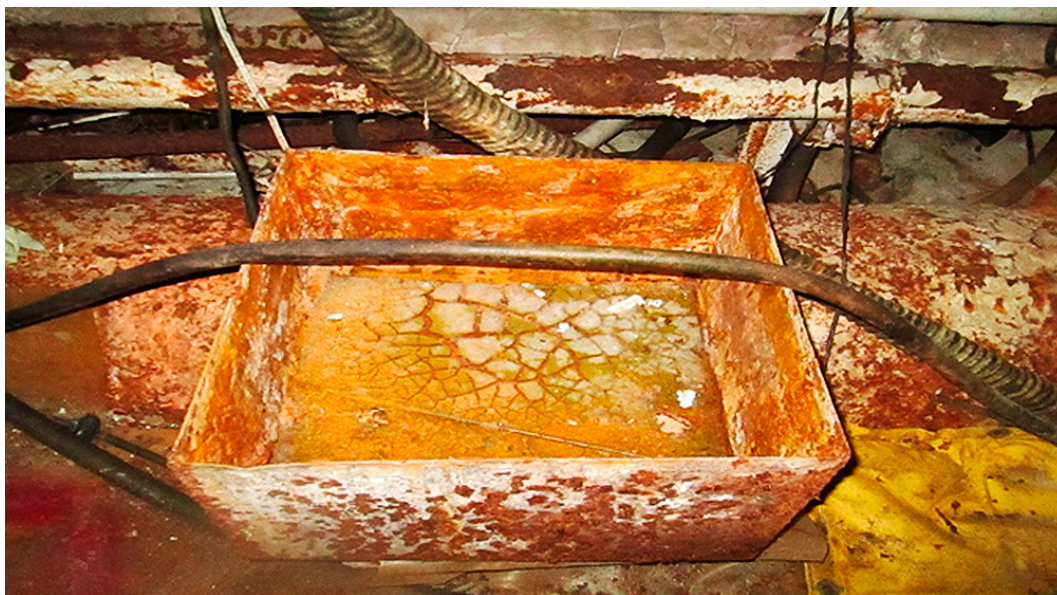
Fig. 3.61 — Radioactive water drying in a container for radioactive water collection from the SDC pipe in room 001/3 of the Shelter object
