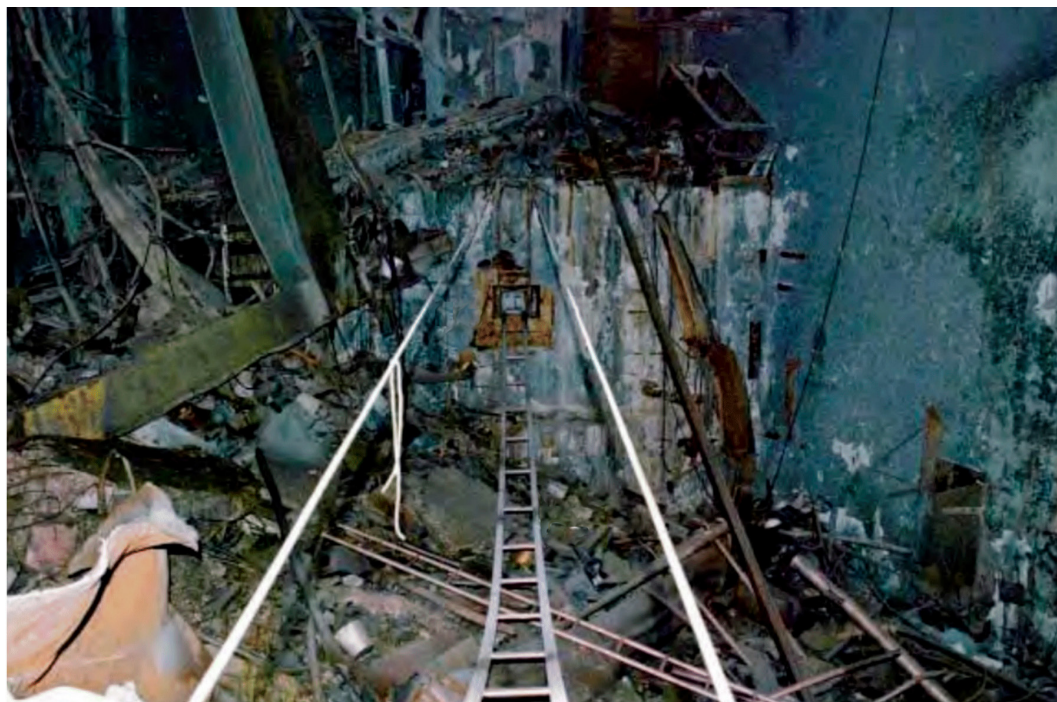
Fig. 2.13 — Transporting of the remote device to the sub-reactor room 305/2 [38]
