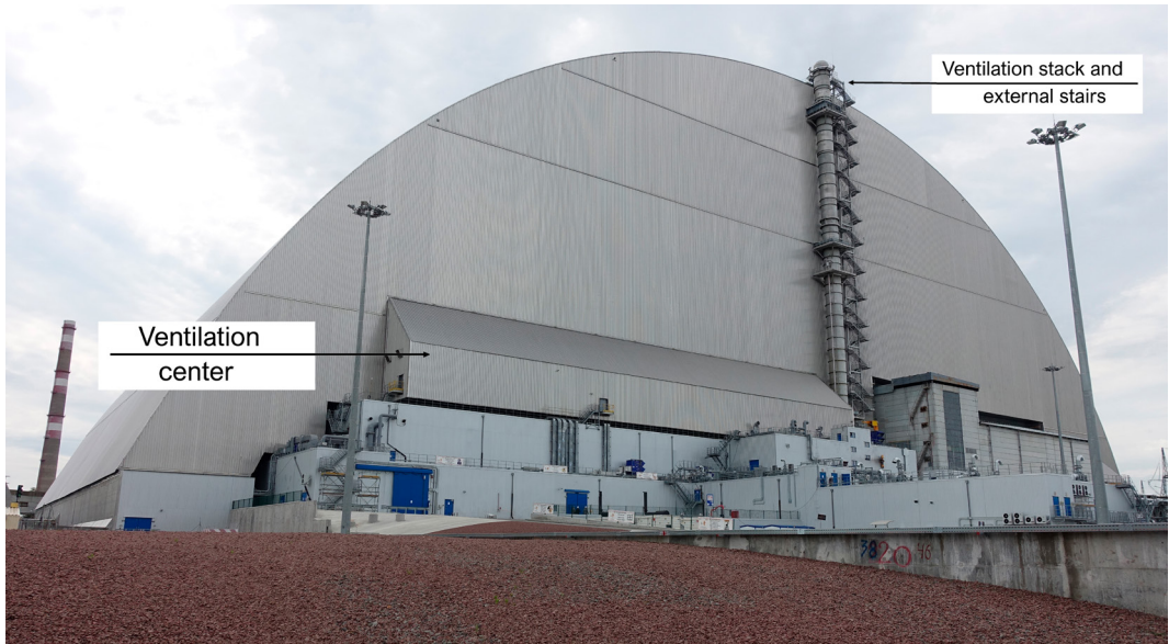
Fig. 1.22 — Structures suspended on the western wall of the arch
