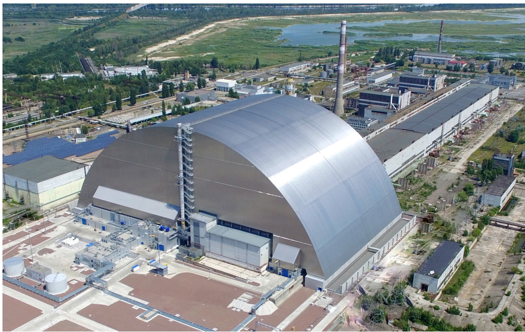
Fig. 1.9 — General view of the NSC after completion of construction
