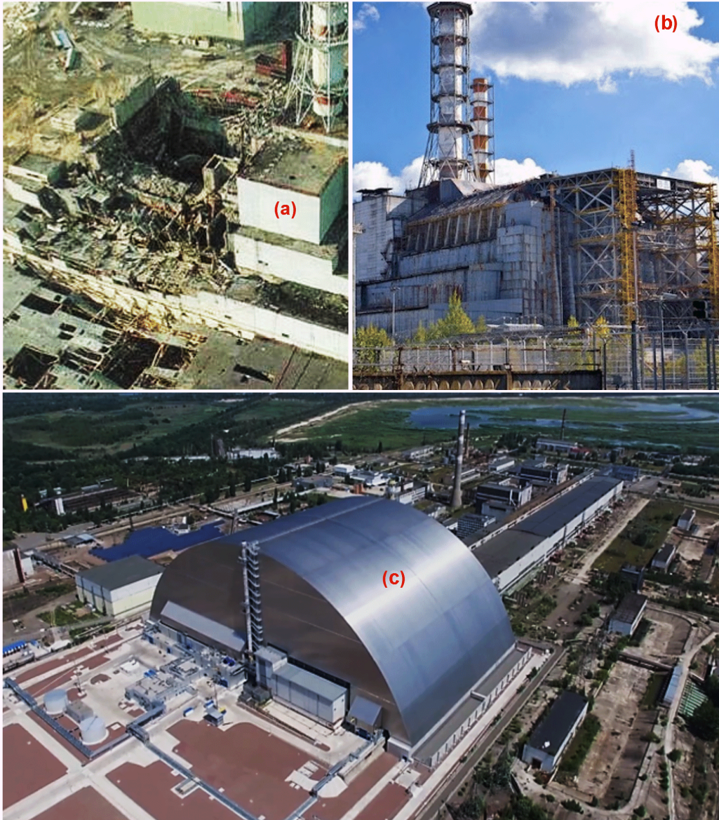
Fig. 2.1 — Transformation of the fourth power unit of the Chornobyl NPP from the accident to the creation of the NSC:
