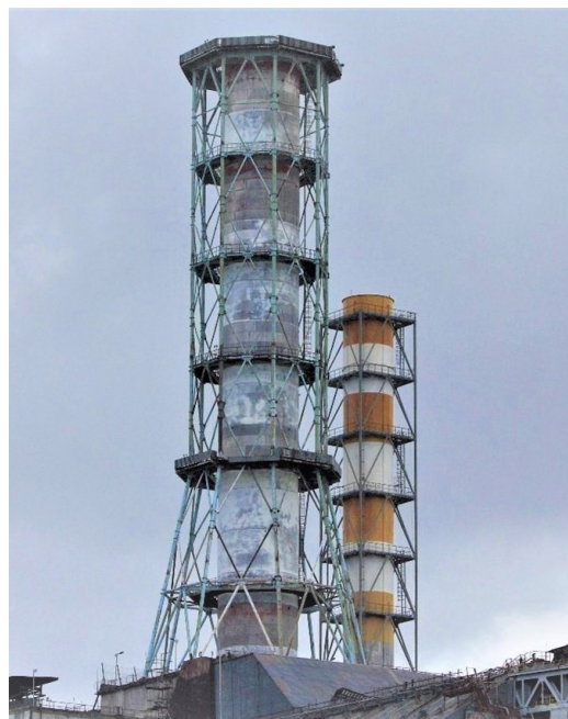
Fig. 1.4 — VT-2 (in the foreground) and new ventilation stack
