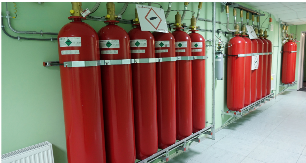
Fig. 1.35 — Automated gas fire extinguishing system
