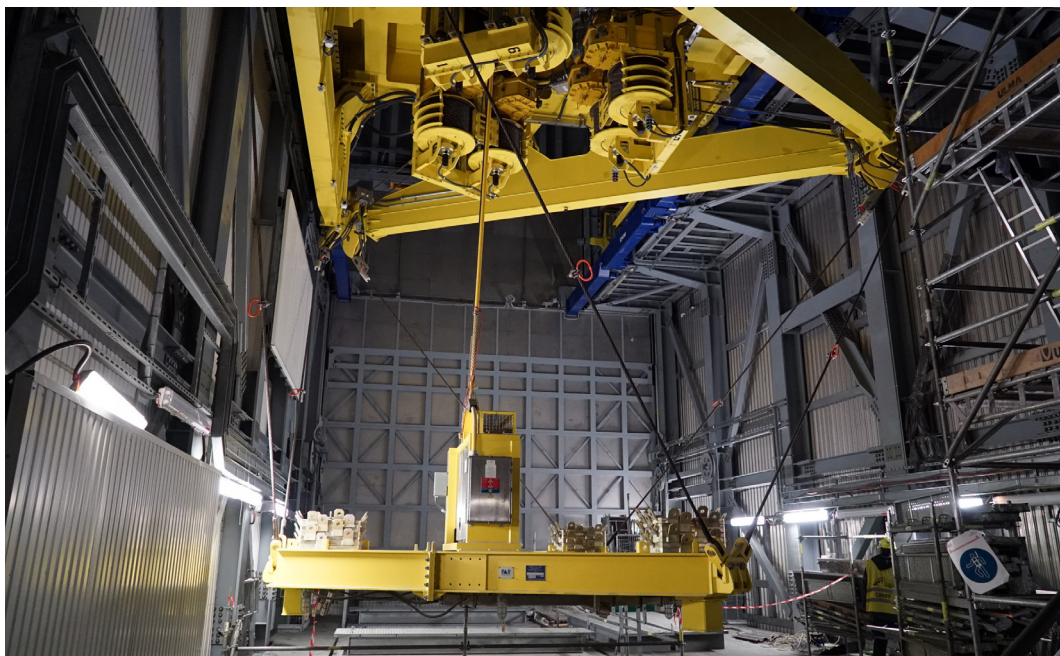
Fig. 1.33 — Maintenance garage with a truck, equipped with a mobile instrumental platform
