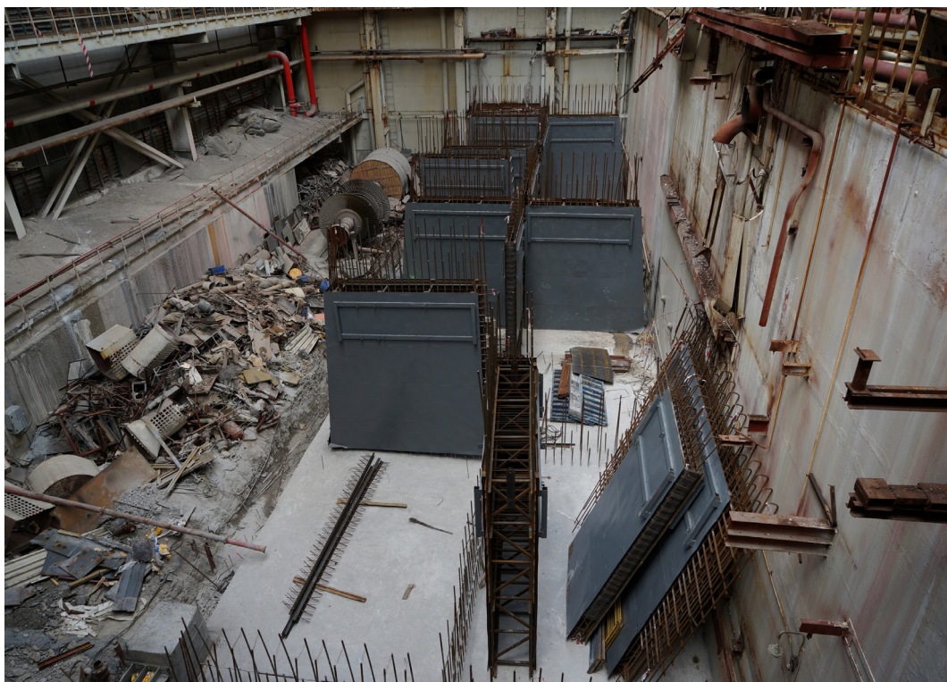
Fig. 1.26 — Construction of the western wall of the NSC EP in the turbine island
