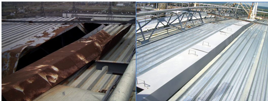
Fig. 3.52 — Replacement of the light roof covering of the Shelter object
