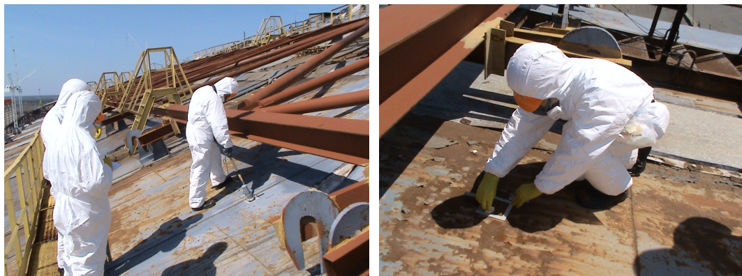
Fig. 6.10 — Measurement of the surface radioactive contamination: a — measurement of the total surface radioactive contamination; b — a sampling of the smear from the area of 10 cm 2
