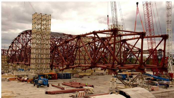
Fig. 1.13 — Erecting the segment of the arch
