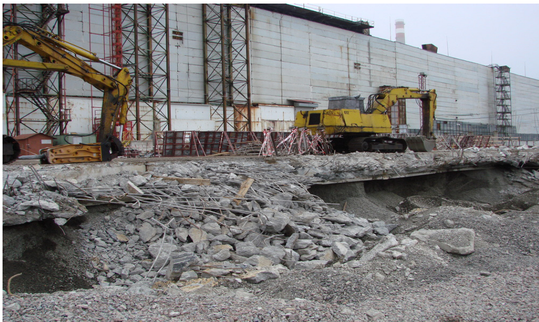
Fig. 1.1 — Disassembly of the pioneer wall berm with a hydrohammer
