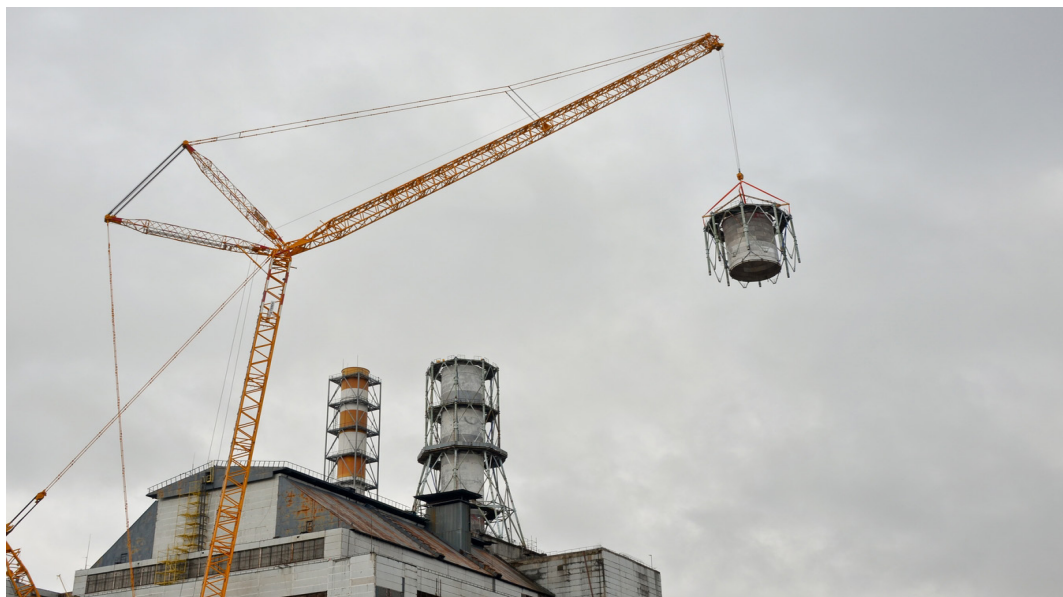
Fig. 1.6 — Dismantling of the intermediate part of the stack trunk with a support platform
