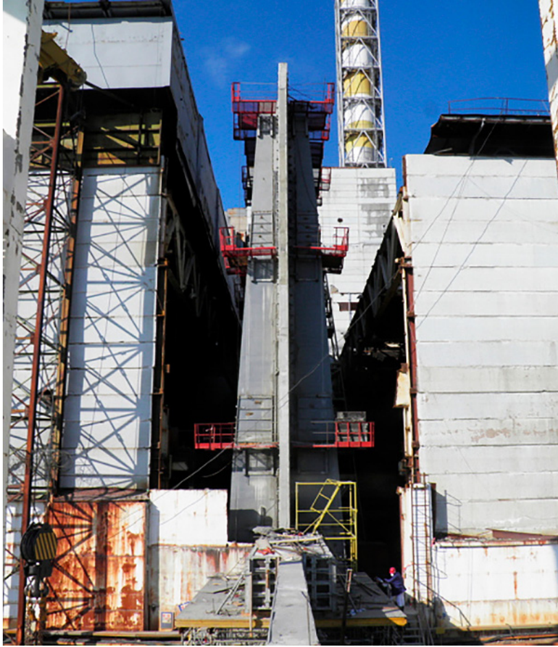
Fig. 1.27 — Eastern end of the NSC enclosing perimeter
