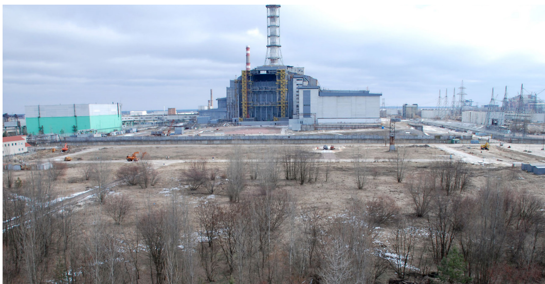
Fig. 1.2 — Preparation of the construction site for the New Safe Confinement
