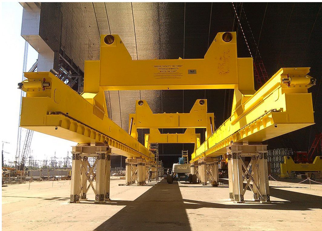
Fig. 1.30 — Construction of a crane bridge prepared for installation on crane girders at the erecting site
