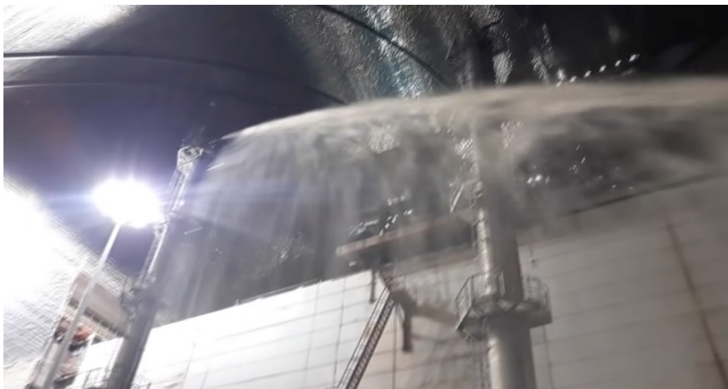
Fig. 1.38 — Testing of the foam fire extinguishing system
