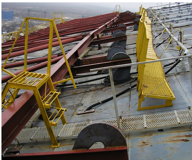
Fig. 6.8 — Assembled metal truss with bridges for the passage to ladders and injectors of the modernized dust suppression system
