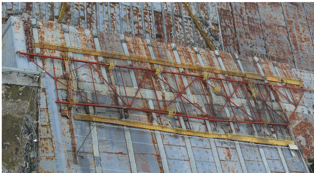
Fig. 6.7 — Metal truss in the design position
