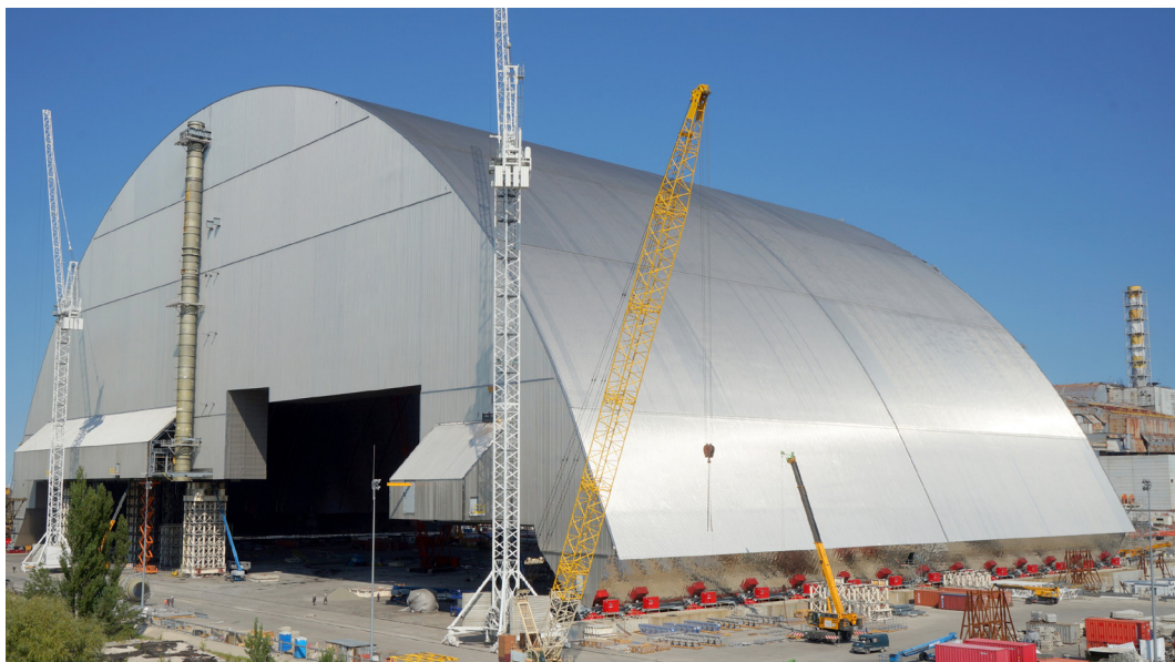
Fig. 1.15 — Arch on the erecting site before it is placed into the design position
